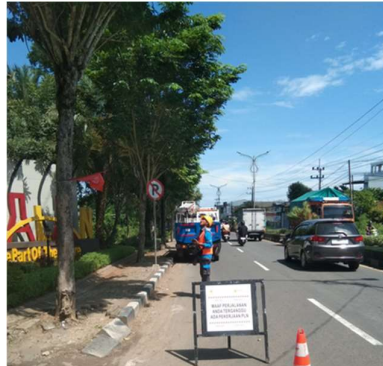
Figure 4. Warning Attention Board
