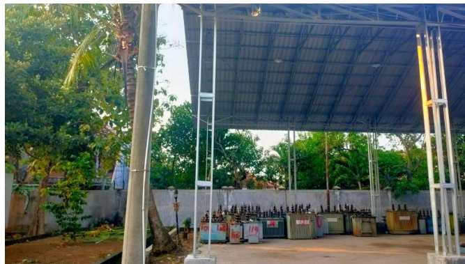
Figure 7. UID Jatim Transformer Warehouse Condition
