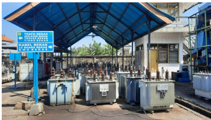
Figure 5. Transformer Warehouse Existing Condition
