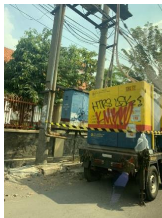
Figure 3. Police Line as a Work Sign
