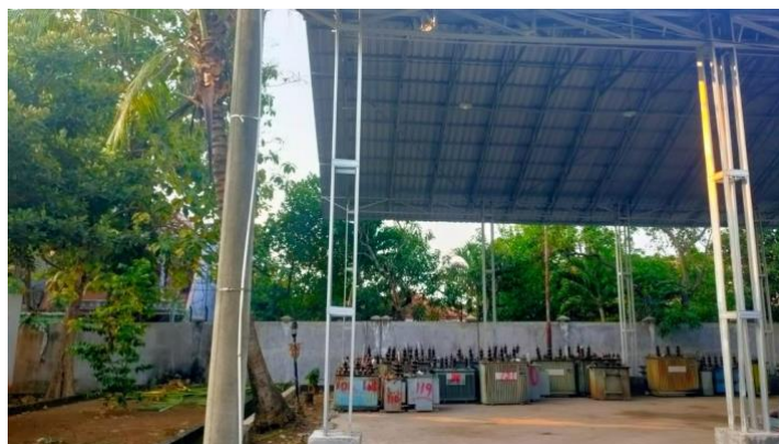
Figure 4. UID Jatim Transformer Warehouse Condition
