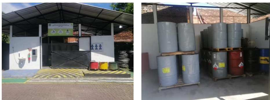
Figure 5. Hazardous Waste Temporary Storage at UP3 Madiun
