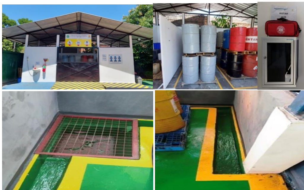
Figure 7. Hazardous Waste Temporary Storage
