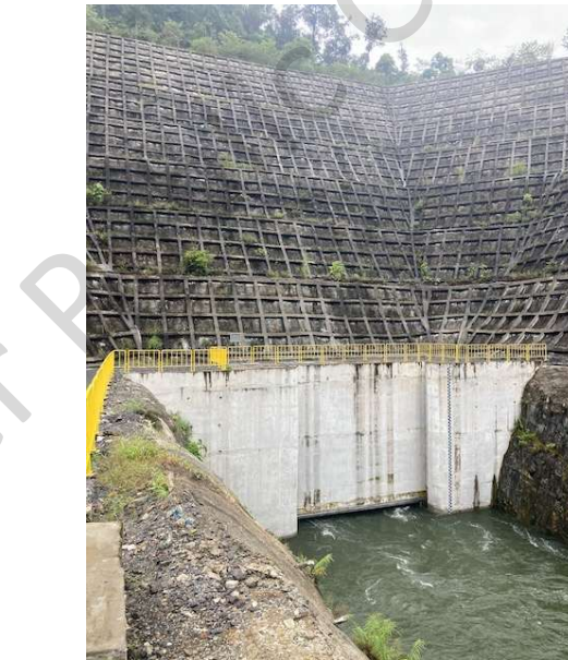
Photo 41: Tailrace tunnel exit
