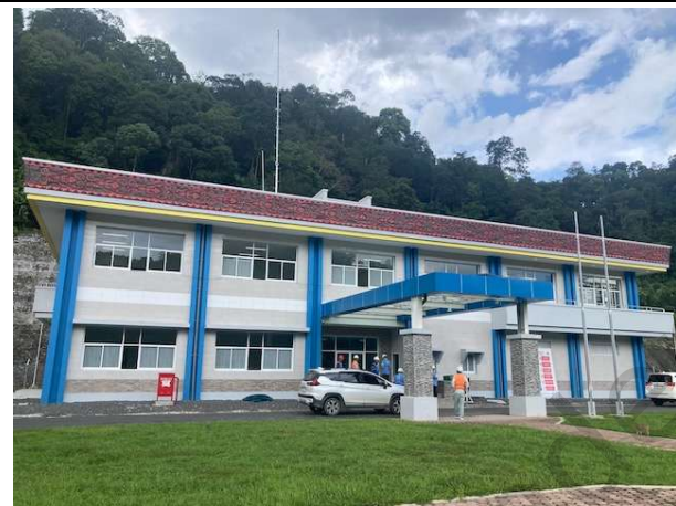
Photo 34: Asahan-3 HPP control and administration building
