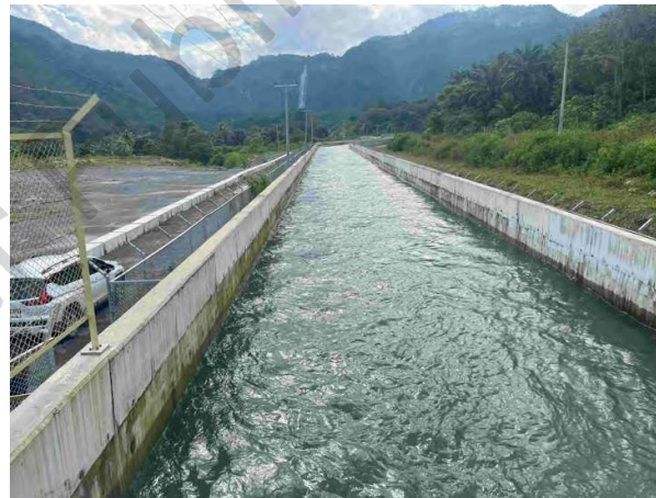
Photo 11: Headrace canal, view towards upstream
