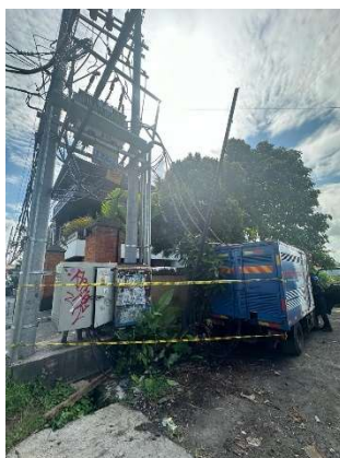
Figure 4. Police Line as a Work Sign
