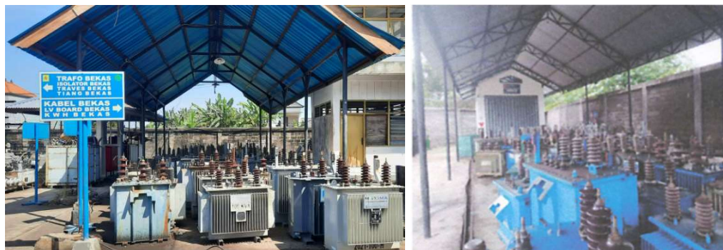
Figure 5. Transformer Warehouse Existing Condition
