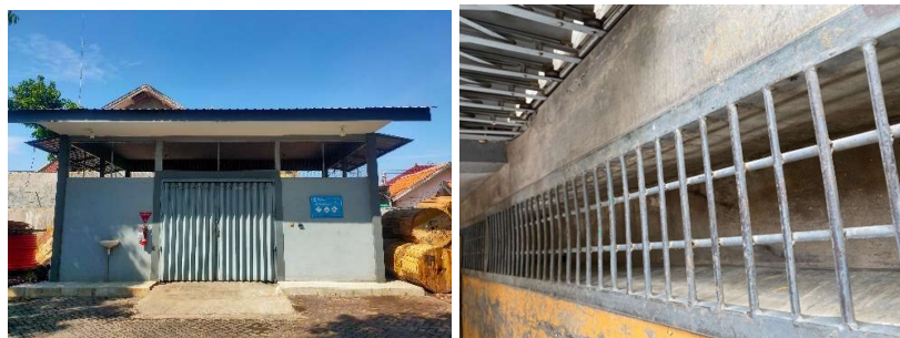
Figure 8. Hazardous Waste Storage at UP3 Pasuruan
